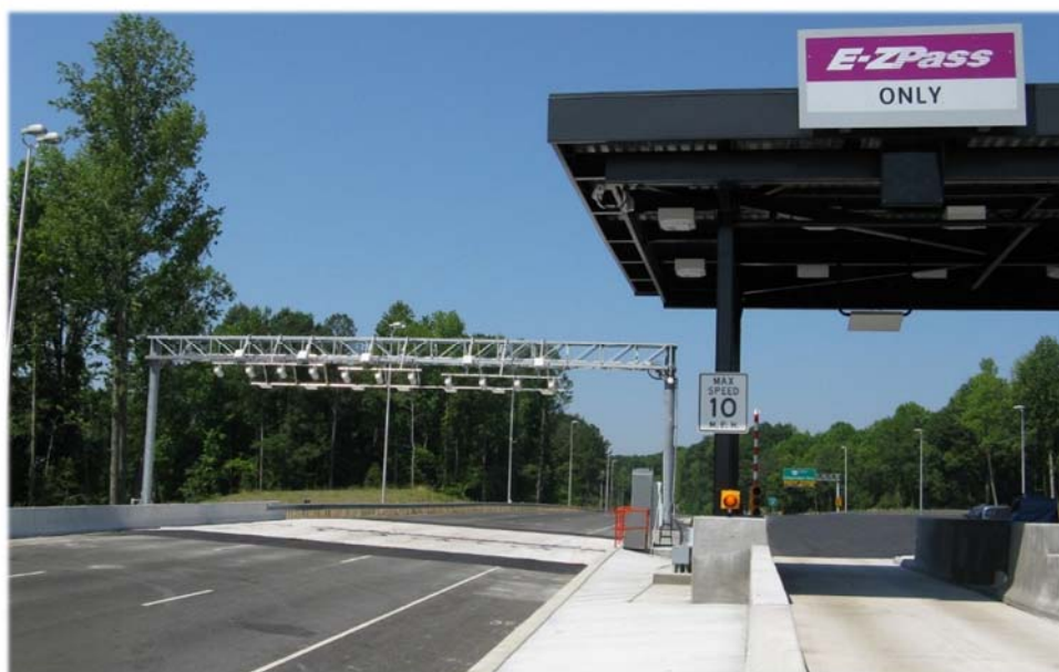
Powhite Parkway Plaza, Express Lanes (left) and Traditional Lanes (right)
