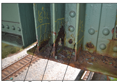
FASCIA STIFFENERS EXISTING CONDITION Partial sections shown. Rivets omitted for clarity Scale: 1/2" = 1'-0"
