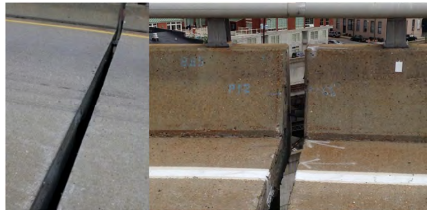
This work includes partial deck removal and reconstruction on the oncoming traffic side of the expansion joint and installation of a preformed elastomeric joint sealer.
