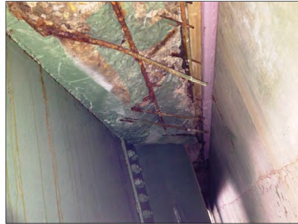
BRIDGE 17 - DECK SOFFIT AT SOUTH ABUTMENT
