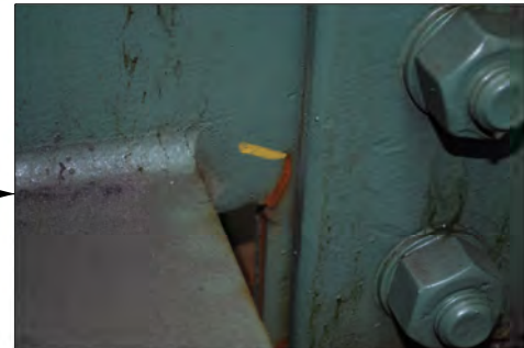
MAGNIFIED VIEW OF CRACK LOCATION
