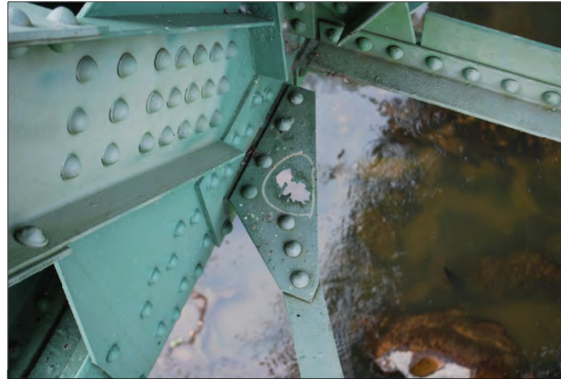
UNIT 12 WEST TRUSS LOWER LATERAL BRACING GUSSET PLATE
