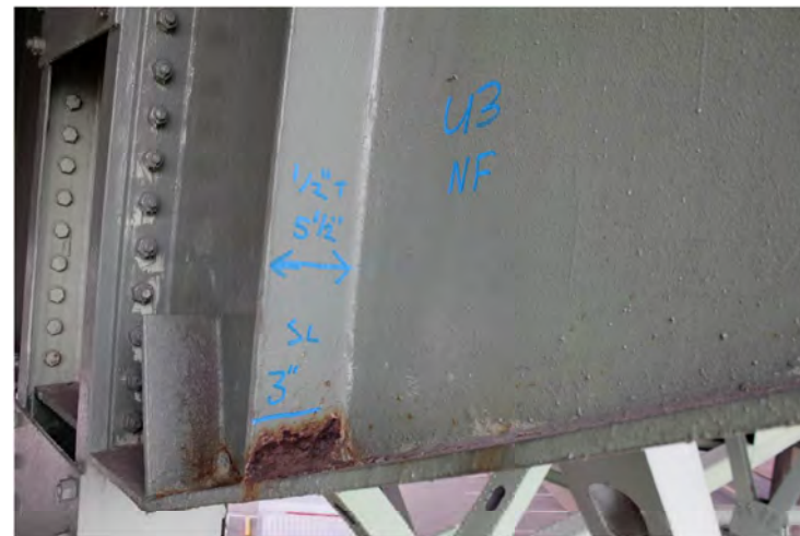
3RD CANTILEVER FLOORBEAM NORTH OF PIER 10W Looking Southeast
