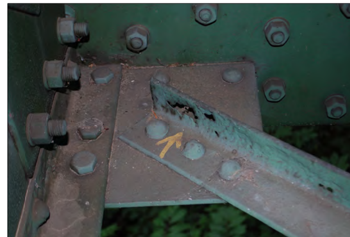
UNIT 15 LATERAL BRACING ANGLE IN EAST TRUSS PANEL POINT 3
