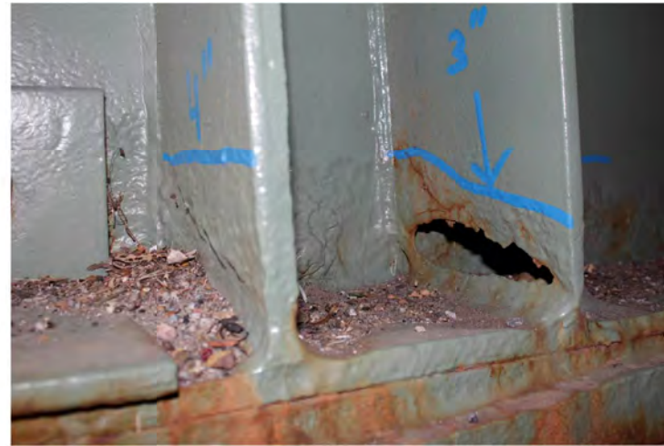
PIER 12W FLOORBEAM 16 STIFFENER PLATE
