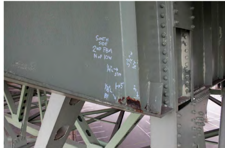
2ND CANTILEVER FLOORBEAM NORTH OF PIER 10W Looking North
