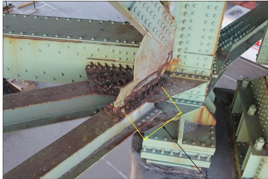
BRIDGE 67, PIER 93-94 LATERAL GUSSET PLATE
