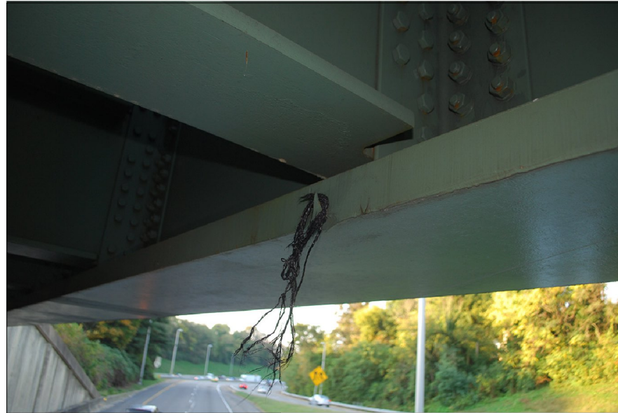
BRIDGE 10S SOUTH GIRDER LOOKING SOUTH
