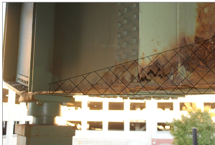
BRIDGE 67, PIER 12W FLOORBEAM 16 LOOKING NORTHWEST
