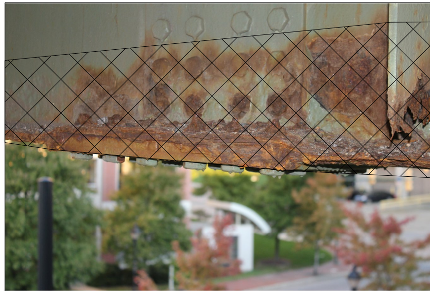
BRIDGE 67, PIER 12W FLOORBEAM 16 LOOKING NORTH
