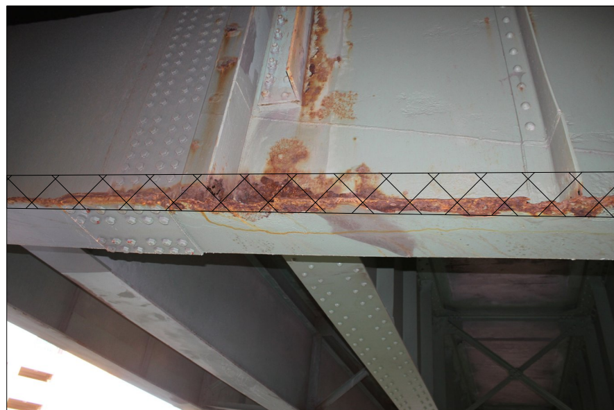
BRIDGE 67, PIER 12W FLOORBEAM 16 LOOKING NORTH
