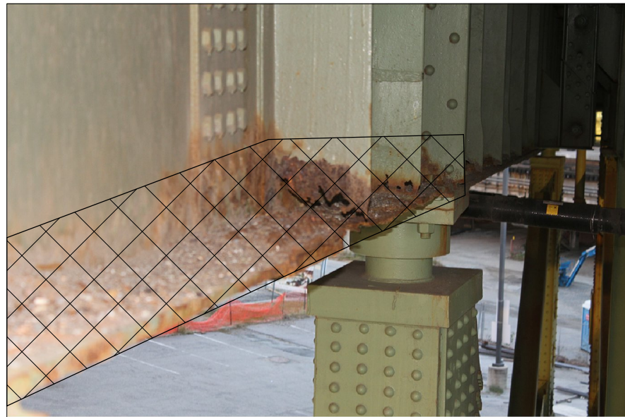
BRIDGE 67, PIER 12W FLOORBEAM 16 LOOKING EAST
