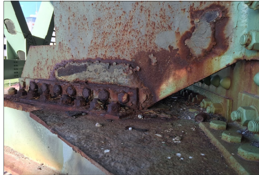
BRIDGE 67, PIER 93-94 LATERAL GUSSET PLATE
