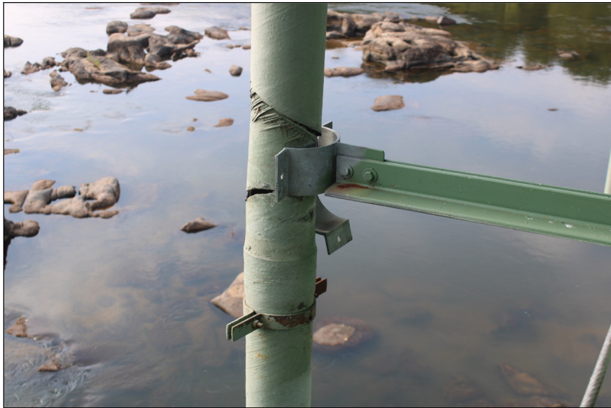
BOULEVARD BRIDGE TYPICAL LOOSE DOWNSPOUT SUPPORT BROKEN DOWNSPOUT
