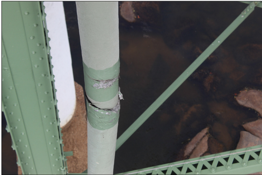
BOULEVARD BRIDGE TYPICAL BROKEN DOWNSPOUT
