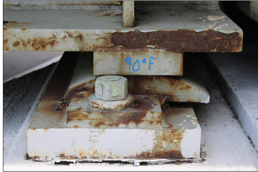
BRIDGE 51 PIER 1, CLOSE UP OF TYPICAL MISALIGNED BEARINGS
