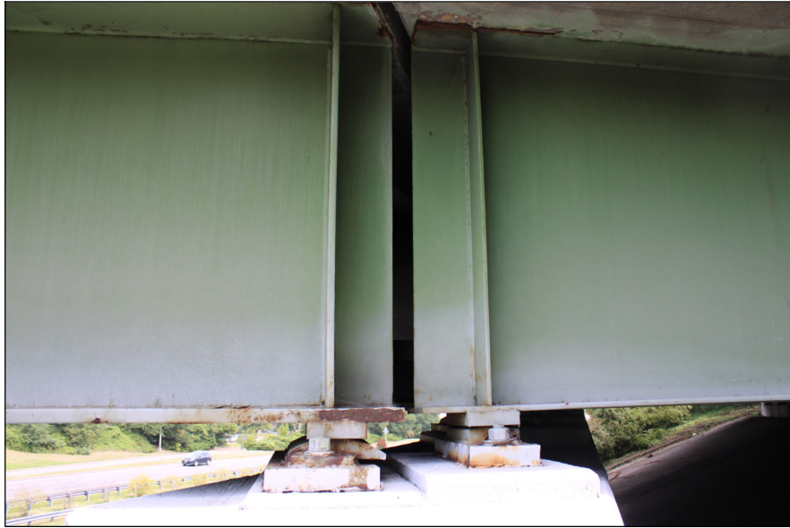
BRIDGE 51 PIER 1, TYPICAL MISALIGNED BEARINGS
