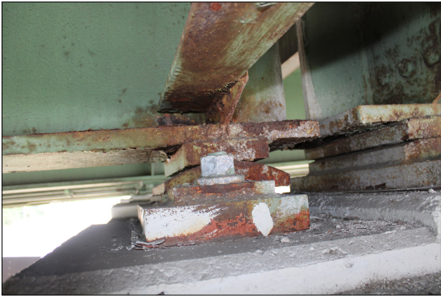
BRIDGE 50 PIER 2, TYPICAL MISALIGNED BEARINGS
