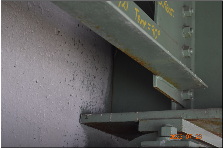
BRIDGE 46 SOUTH ABUTMENT TYPICAL JAMMED GIRDER END
