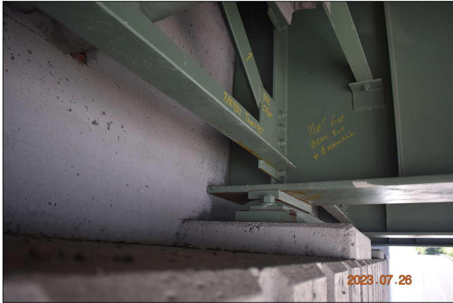
BRIDGE 46 SOUTH ABUTMENT TYPICAL MISALIGNED BEARING
