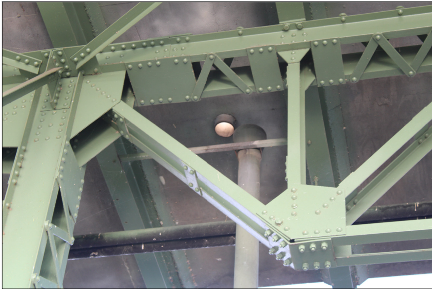
BOULEVARD BRIDGE TYPICAL MISALIGNED DOWNSPOUT
