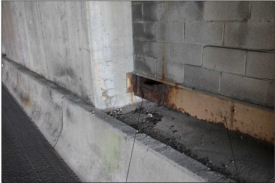
AREA OF SECTION LOSS
