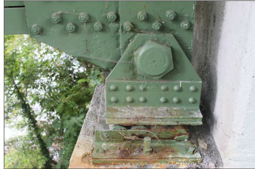
BOULEVARD BRIDGE TYPICAL EXPANSION BEARING CONDITION
