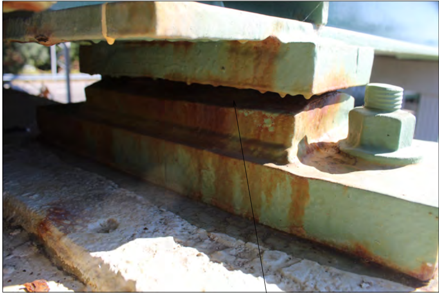
REMOVE ACCESSIBLE PACK RUST AND SEAL
