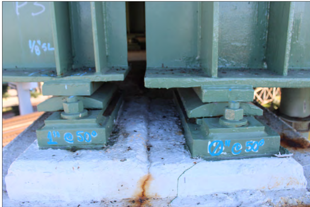
BRIDGE 68 PIER 3, UNIT 6 TYPICAL MISALIGNED BEARING
