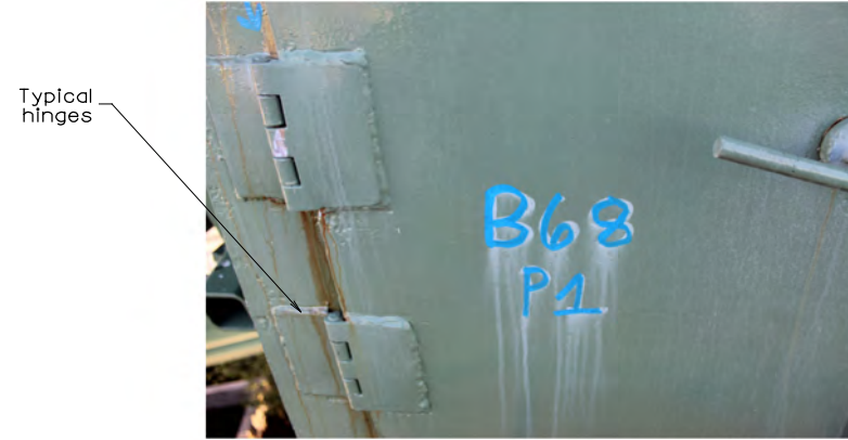
BRIDGE 68 PIER 1 - TYPICAL DOOR HINGES
