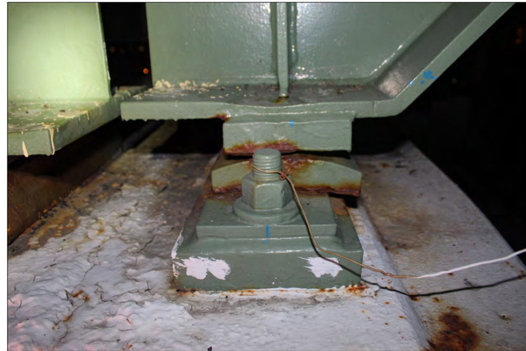
BRIDGE 68 PIER 5, UNIT 8 TYPICAL MISALIGNED BEARING
