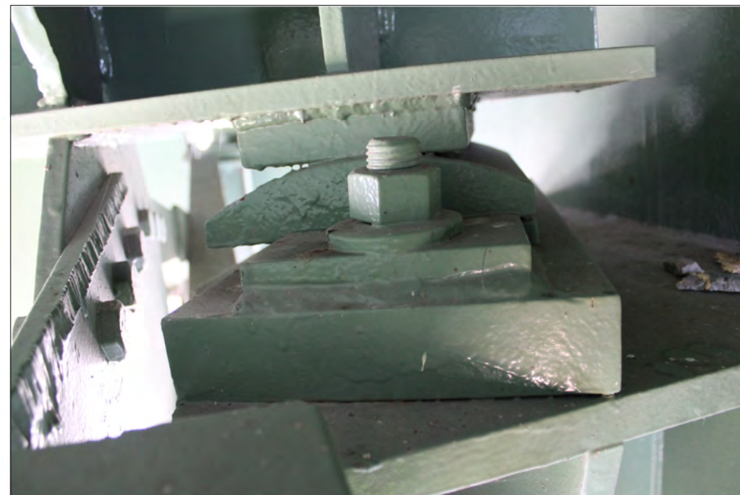
BRIDGE 68 PIER 20, UNIT 1 TYPICAL MISALIGNED BEARING
