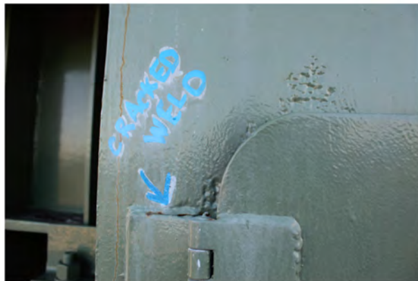
BRIDGE 68 TYPICAL DOOR HINGE CRACKED WELD
