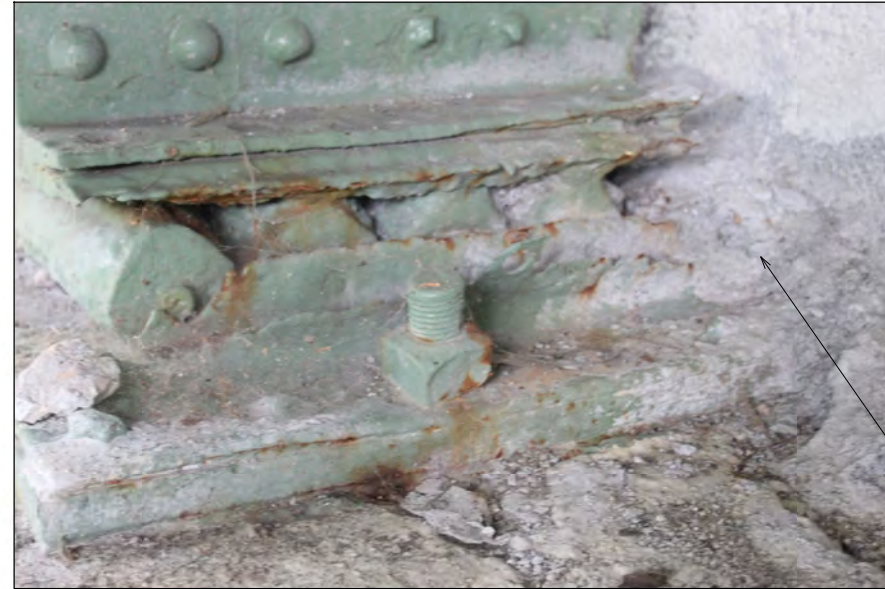
BOULEVARD BRIDGE PIER 27 WEST TRUSS BEARINGS CONCRETE DEBRIS
