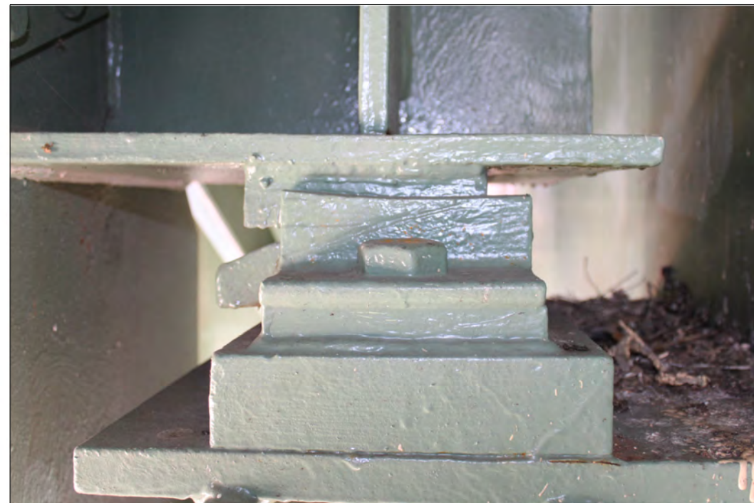
BRIDGE 66 TYPICAL MISALIGNED BEARING LOCATED AT CROSS BOX PIER CAP
