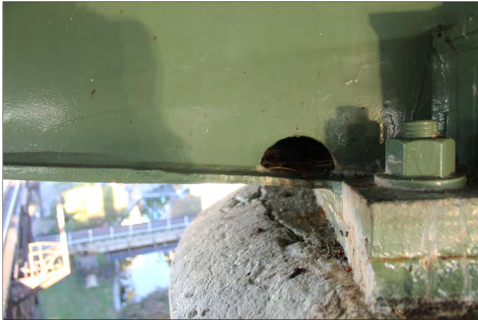
BRIDGE 68 PIER 1 - TYPICAL DRAIN HOLE
