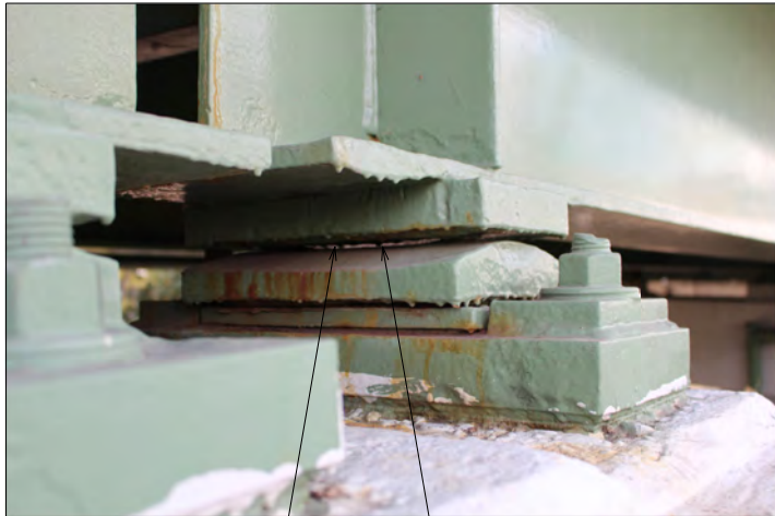
BRIDGE 66 PIER 3 TYPICAL PACK RUST BETWEEN BEARING AND SOLE PLATE
