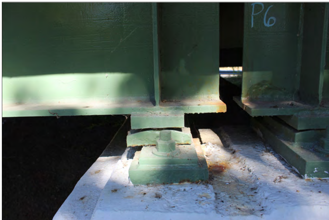
BRIDGE 66, PIER 6 TYPICAL MISALIGNED BEARING
