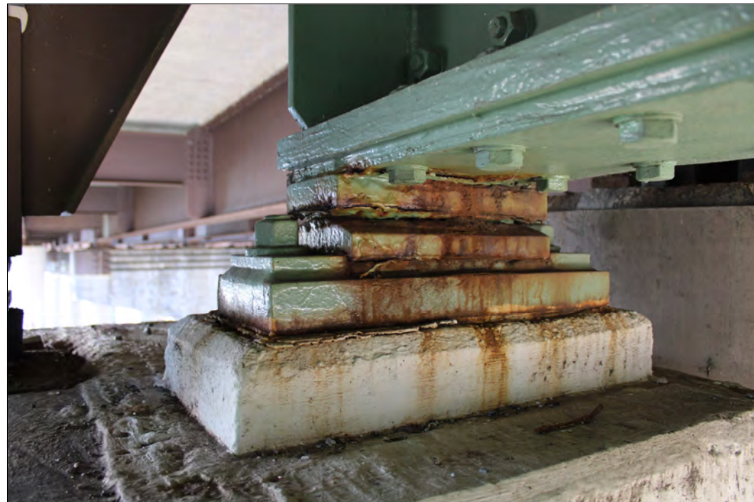
BRIDGE 65 PIER 4 TYPICAL MISALIGNED BEARING WITH PACK RUST
