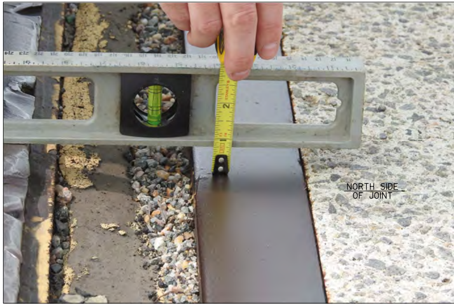
TYPICAL UNLEVEL DECK JOINT
