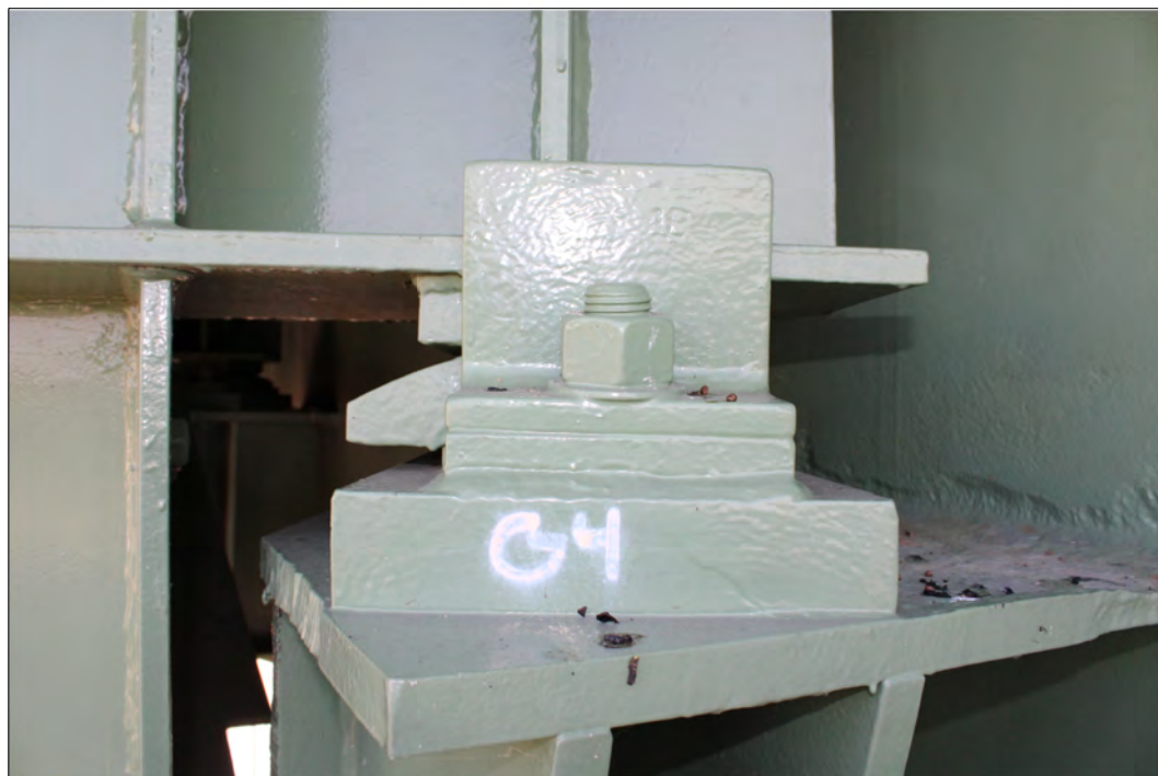
BRIDGE 68 PIER 20, UNIT 1 TYPICAL MISALIGNED BEARING
