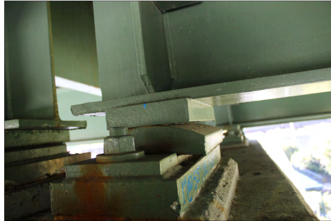
BRIDGE 66, PIER 13 TYPICAL MISALIGNED BEARING
