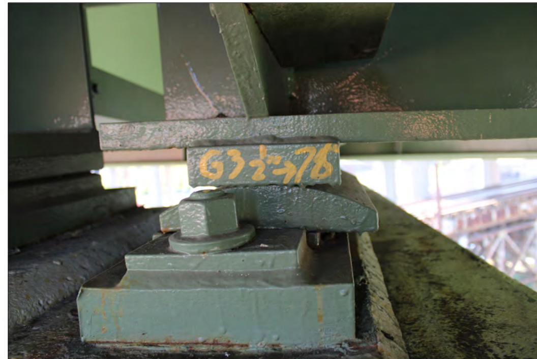
BRIDGE 65 PIER 14 TYPICAL MISALIGNED BEARING
