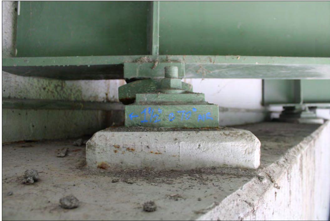
BRIDGE 66 WEST ABUTMENT TYPICAL MISALIGNED BEARING
