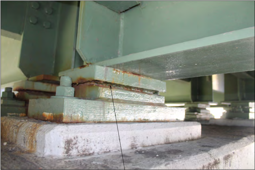
REMOVE ACCESSIBLE PACK RUST AND SEAL
