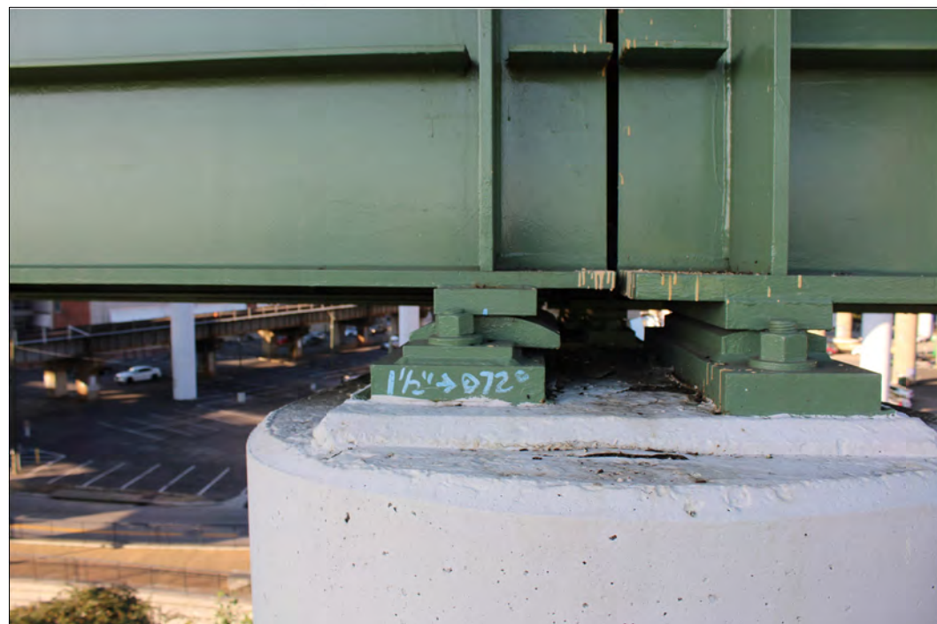
BRIDGE 65 PIER 18 TYPICAL MISALIGNED BEARING
