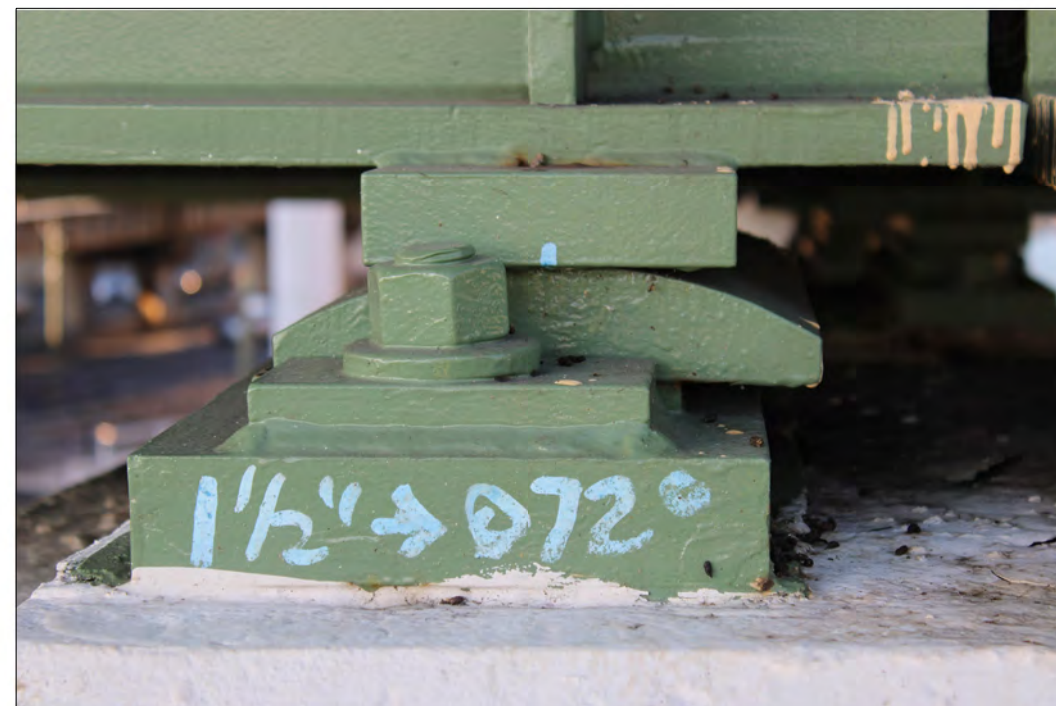
BRIDGE 65 PIER 18 CLOSE-UP OF TYPICAL MISALIGNED BEARING
