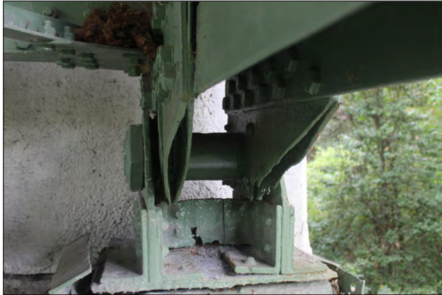
BOULEVARD BRIDGE PIER 27 BEARING EAST BEARING CONDITION
