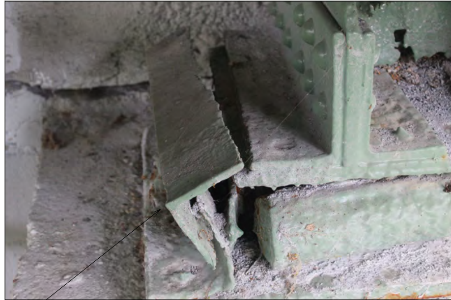
BOULEVARD BRIDGE PIER 27 - BEARING EXISTING KEEPER ANGLE CONDITION
