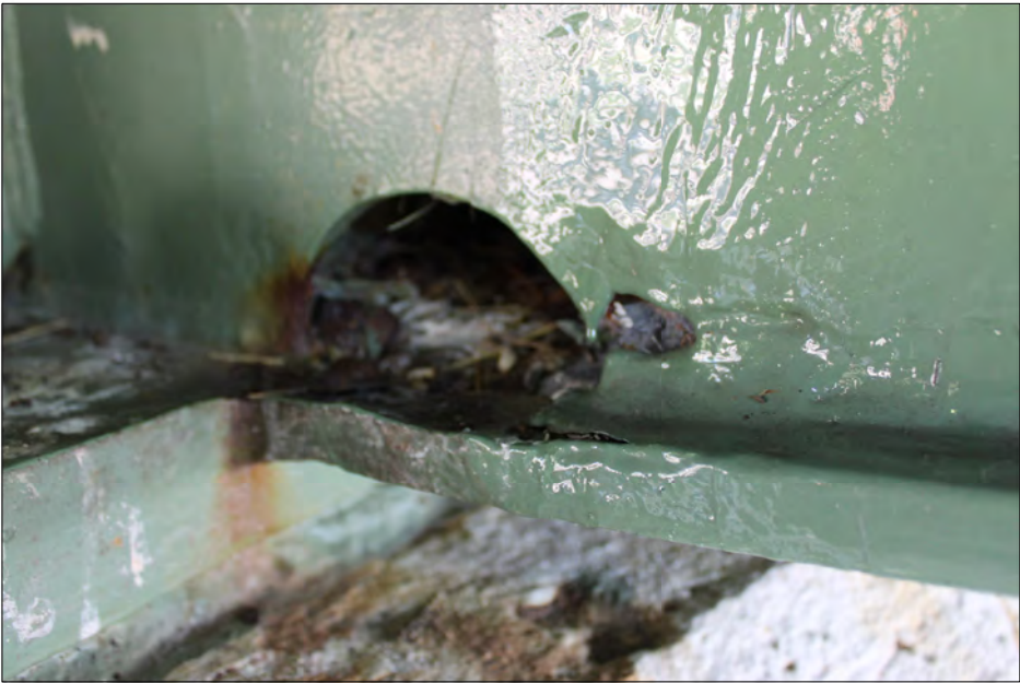
BRIDGE 68 PIER 2 - TYPICAL DRAIN HOLE
