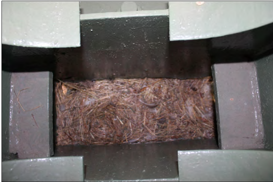
BRIDGE 68 PIER 1 - TYPICAL DEBRIS ACCUMULATION
