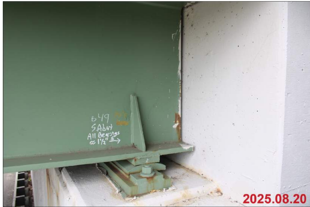
BRIDGE 49 SOUTH ABUTMENT TYPICAL MISALIGNED BEARING
