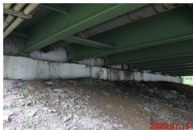
BRIDGE 8N, ABUTMENT 2
