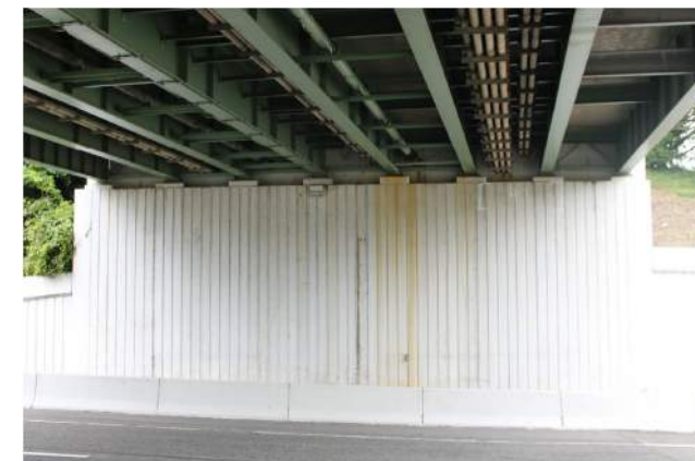
BRIDGE 48, ABUTMENT 2 (LOOKING NORTH)
