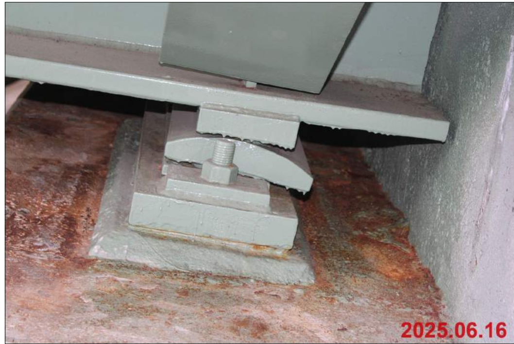
BRIDGE 56 SOUTH ABUTMENT TYPICAL MISALIGNED BEARING
