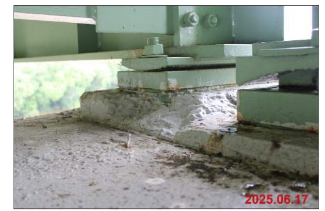
TYPICAL BEARING PEDESTAL SPALL
