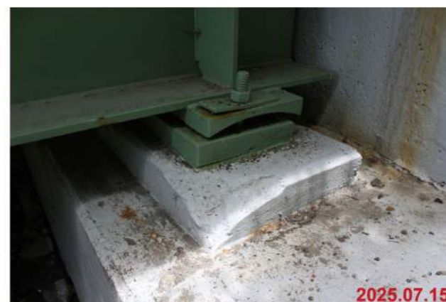
BRIDGE 8N, ABUTMENT 2
