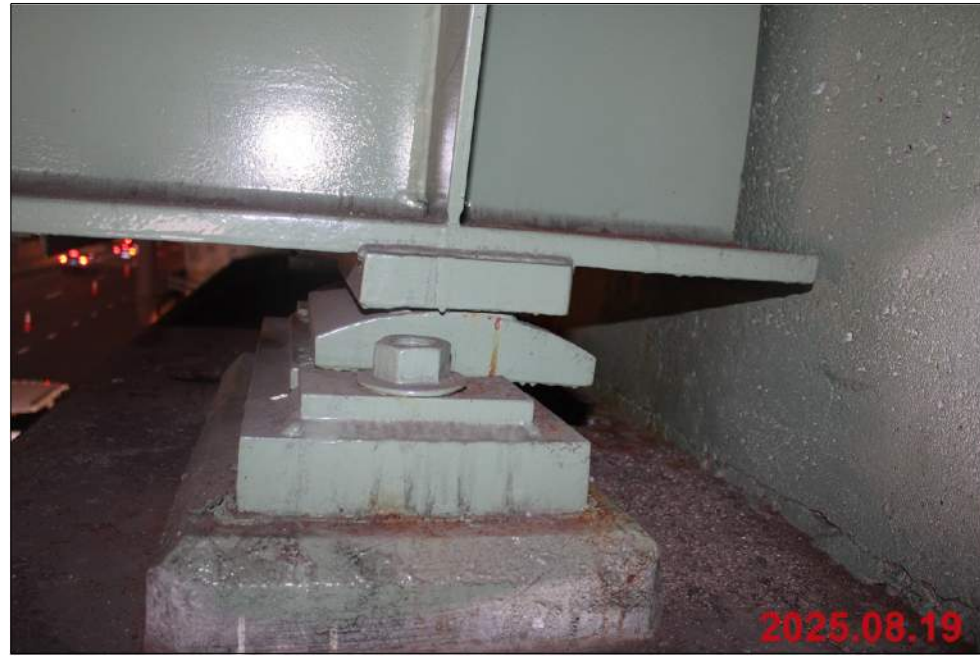
BRIDGE 60 NORTH ABUTMENT TYPICAL MISALIGNED BEARING
