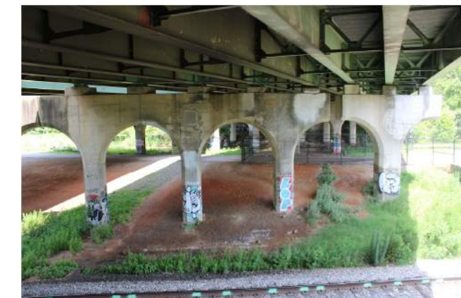
TYPICAL B8N LAND PIER CONDITION
