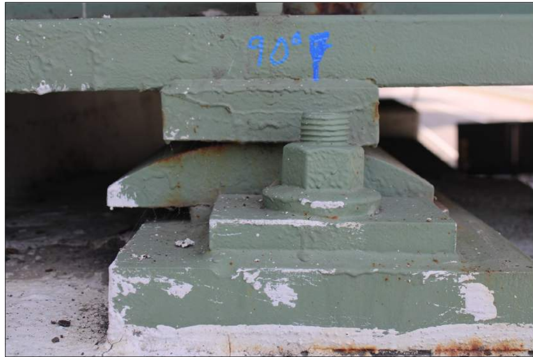
BRIDGE 48 SOUTH ABUTMENT TYPICAL MISALIGNED BEARING
