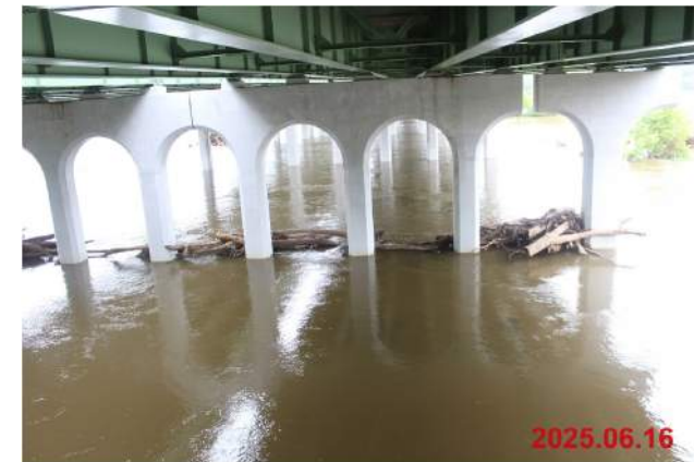
TYPICAL B8N WATER PIER CONDITION
